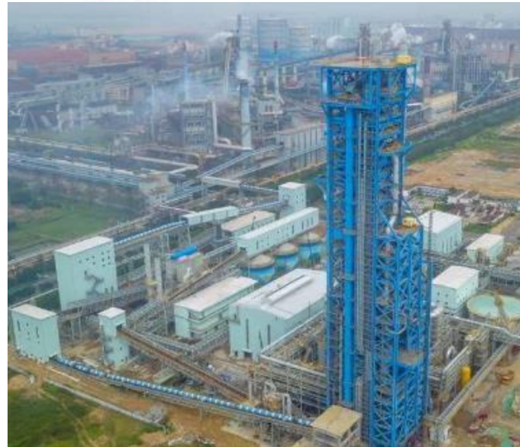
Second DRI Plant in China 1,000,000 tpy DRI Flexible to use diff. gases, including H 2
