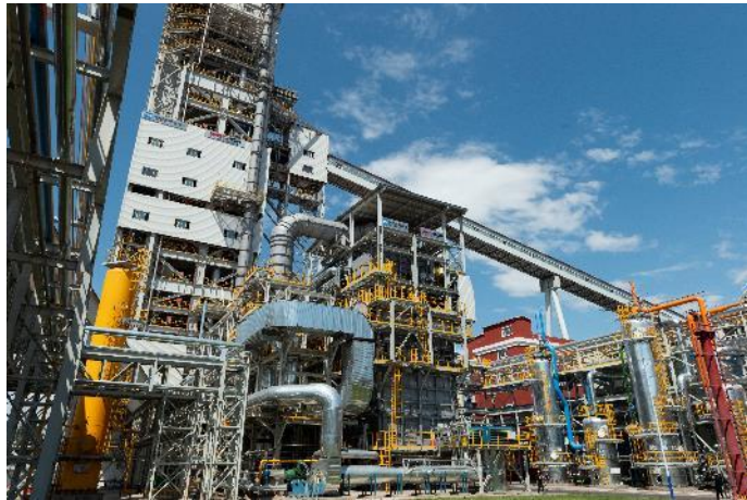
First DRI Plant in China 550,000 tpy DRI 70%H 2 in makeup gases
