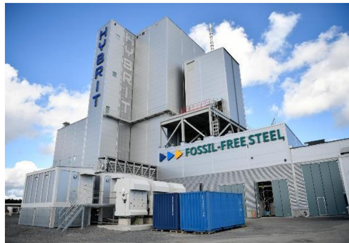
H 2 -based DRI Pilot Plant
