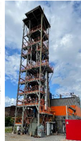
μDRAL Plant operating with NG/H 2
