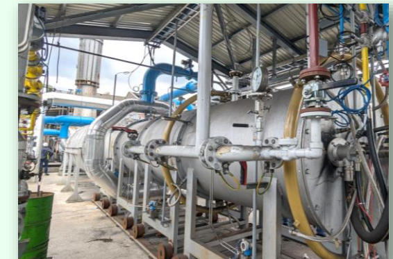
Pilot installation for by-products valorisation
